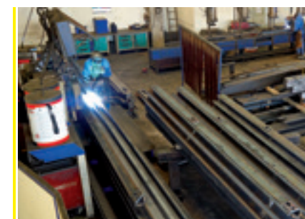
longitudinal welding station
