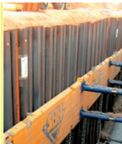
Pile chamber plates h = 1.00\text{ m}
